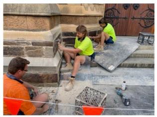
In the past year, we successfully applied for a Heritage SA grant providing matched funding up to an amount of \$20,000 for conservation of stonework on the Pennington Terrace frontage, including the removal of unsuitable or deteriorated mortar, stone repairs, cleaning of stonework, and stripping and repainting of metal work. The cost of this project is around
