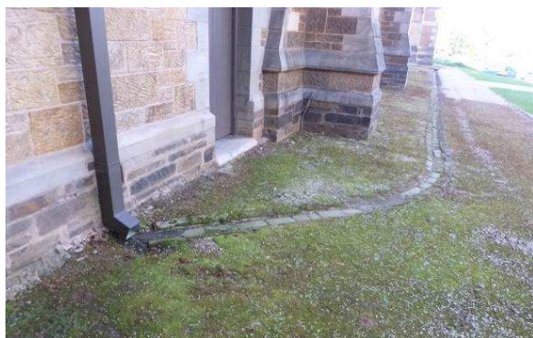
Details of base of South Elevation showing downpipes discharging water on the ground, causing damp ground
