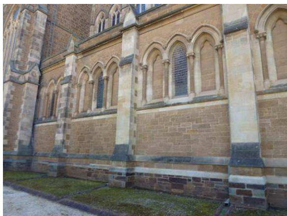
Base of South Elevation - downpipes discharging water into brick drains
