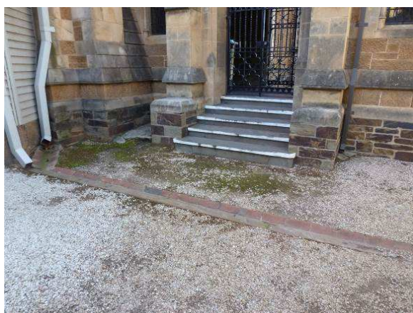
Base of South Elevation - downpipes discharging water into brick drains
