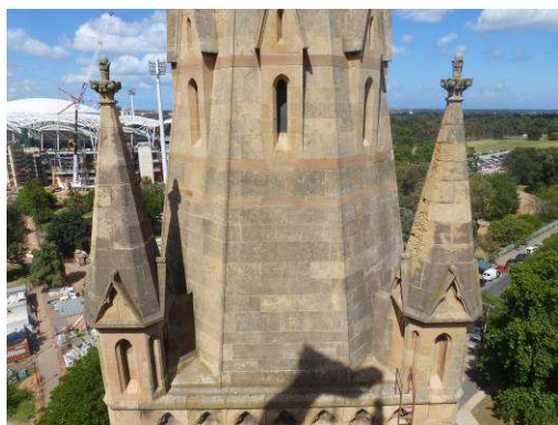
Spire, showing deteriorated limestone (arrowed) and banding of Pyrmont Stone
