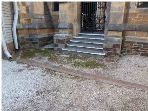
Base of South Elevation - steps to porch (left) and downpipes discharging water into brick drains
