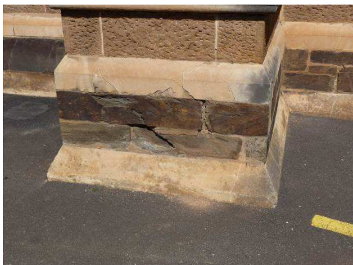
Glen Osmond Bluestone Plinth, with limestone banding (North Elevation, Bay E2 – note deterioration)
