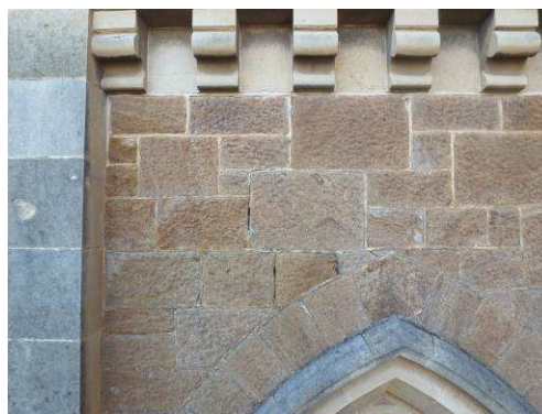
Sandstone to the nave walls, with limestone dressings (extension of nave undertaken in 1890 – 94)
