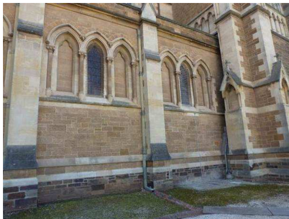
Base of South Elevation - steps to porch (left) and downpipes discharging water into brick drains
