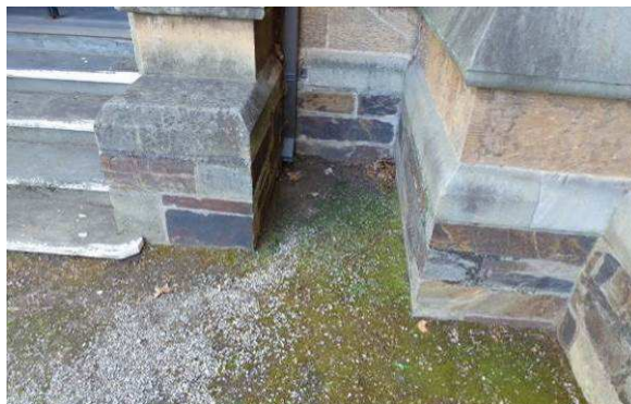
Details of base of South Elevation showing downpipes discharging water on the ground, causing damp ground
