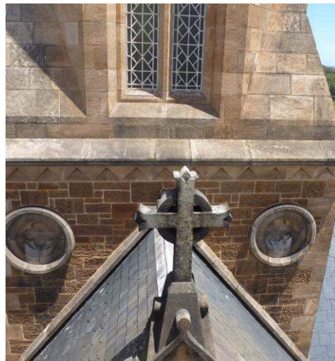
Sandstone to the crossing tower, with sandstone dressings (early 1869 section of Cathedral), note stone cross
